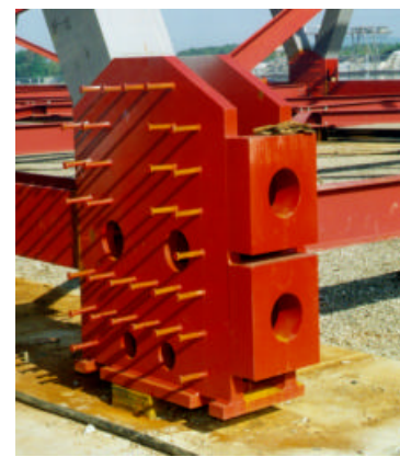
Fig. 10 Node at abutment
