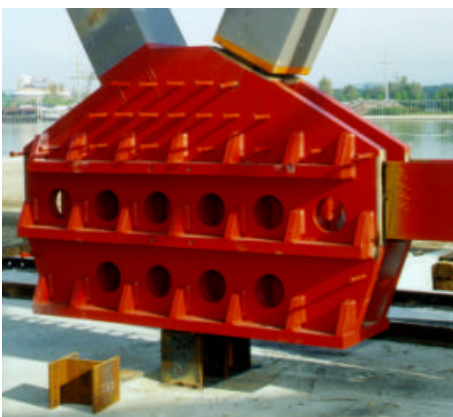
Fig.8 Node at pier
