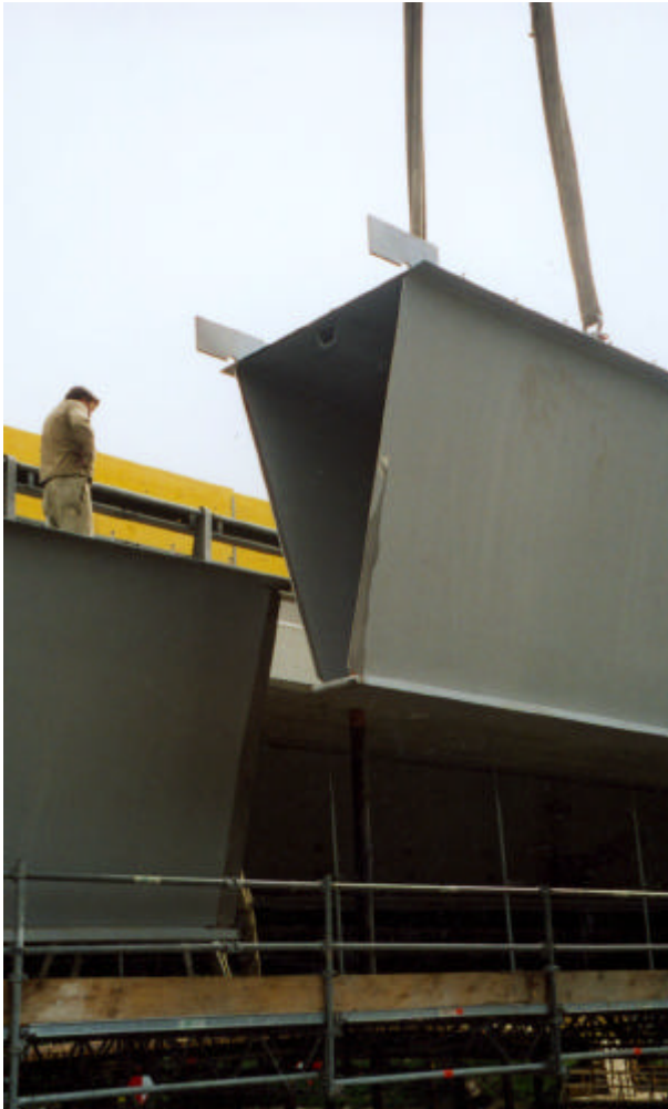
Figure 9: Positioning of the girder
