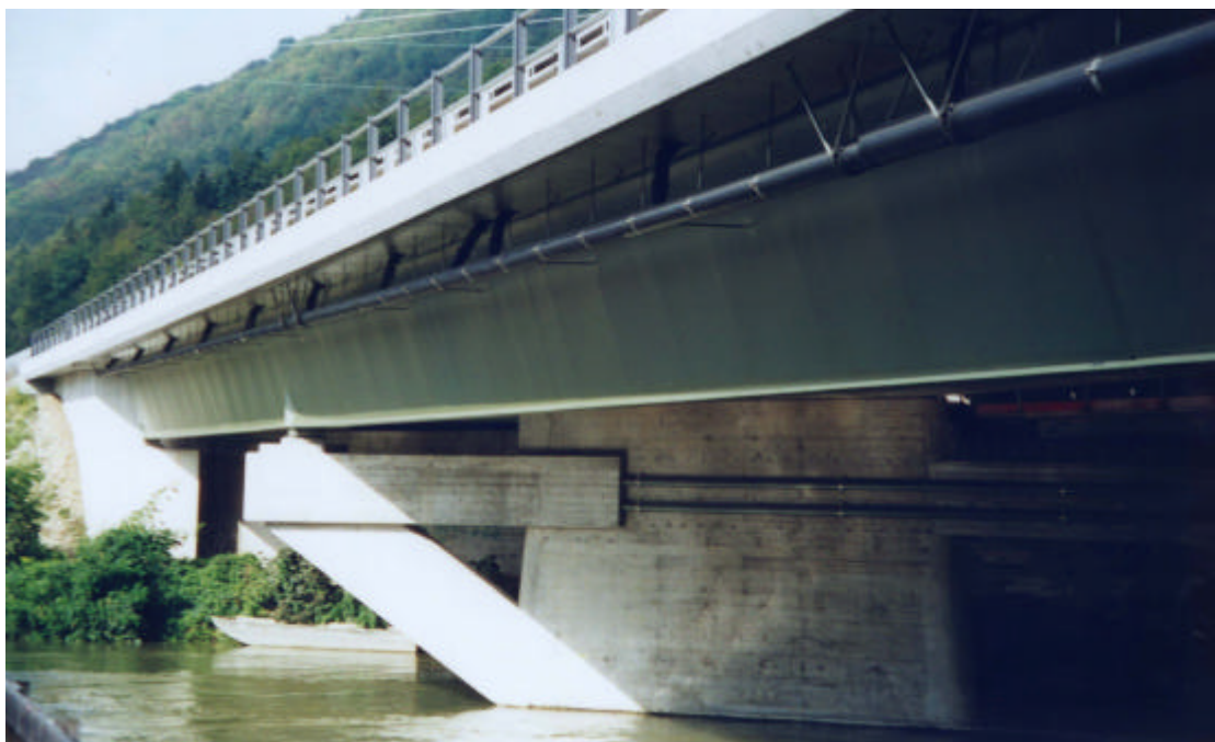
Figure 7: New support at the pier
