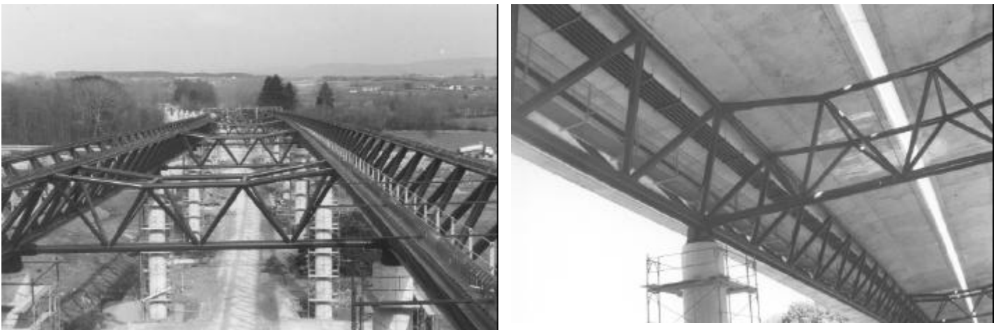
Fig 6 and 7 Brace truss during erection and after completion
